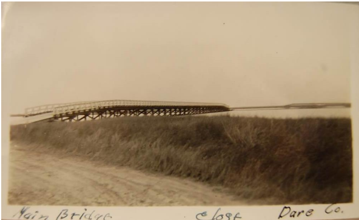
Figure 11. North Channel Bridge: caption reads “Main Inlet Bridge close Dare Co.” (State Highway Commission, ca.1935)
