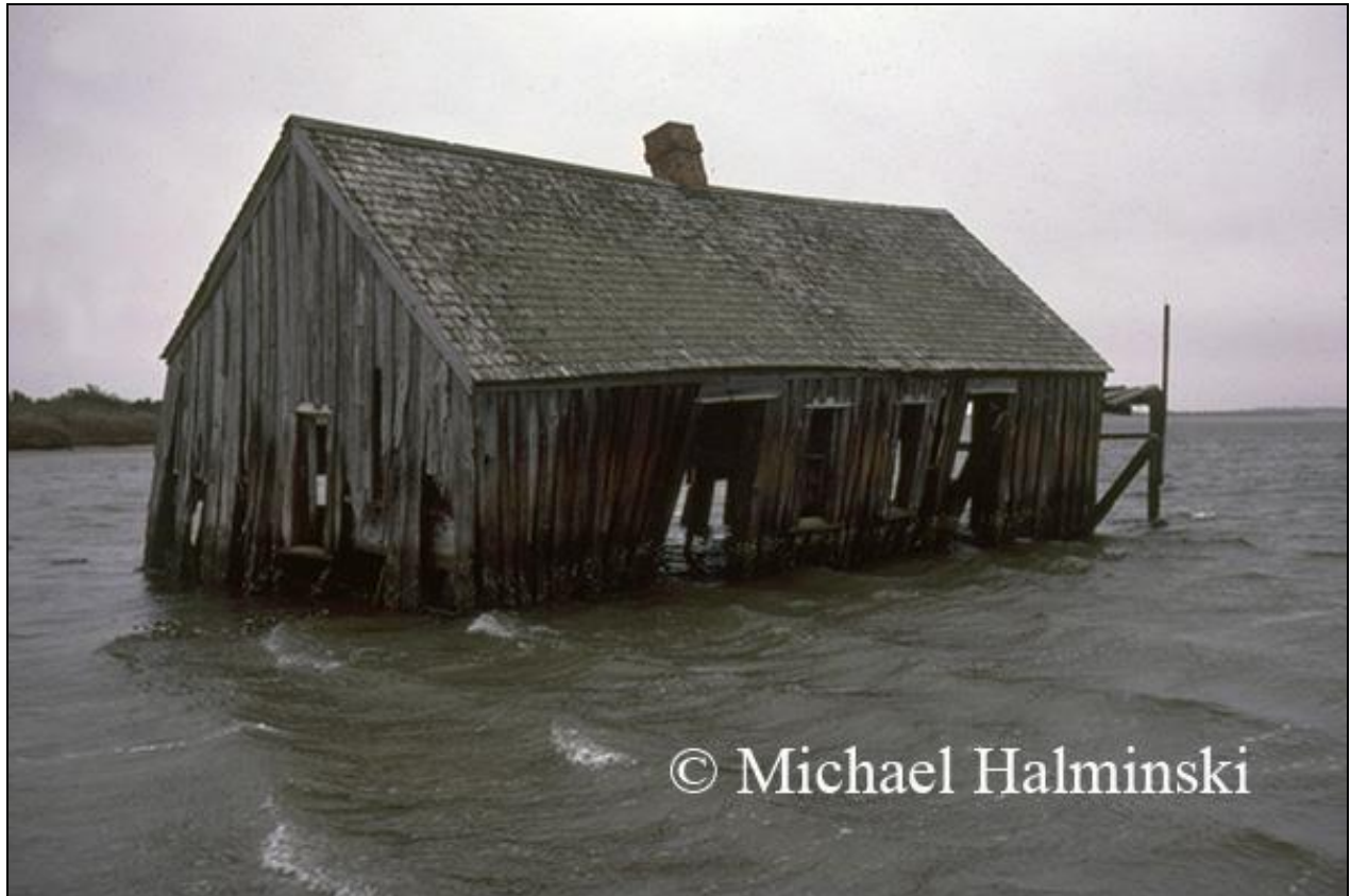
Figure 22. St. Clair Midgett fish camp building off its foundation in the water (photographer: Michael Halminski, January 1985)
