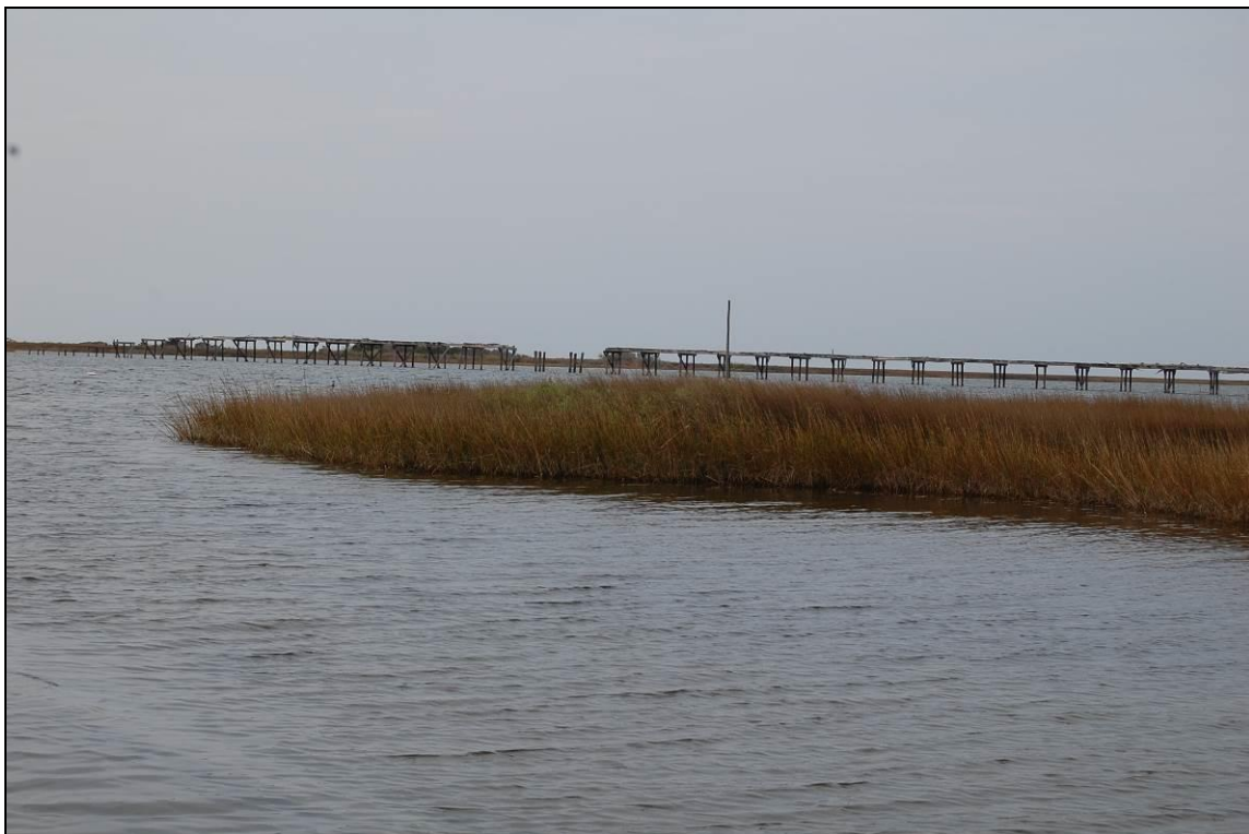
Figure 29. Southern and central sections of North Channel Bridge from NC 12 (photographer: Marvin Brown, November 9, 2016)
