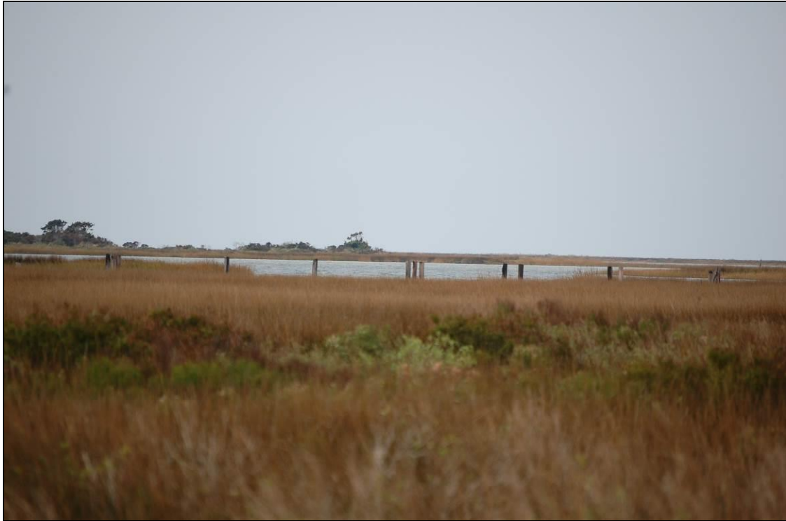
Figure 30. Northern section of North Channel Bridge from NC 12 (photographer: Marvin Brown, November 9, 2016)
