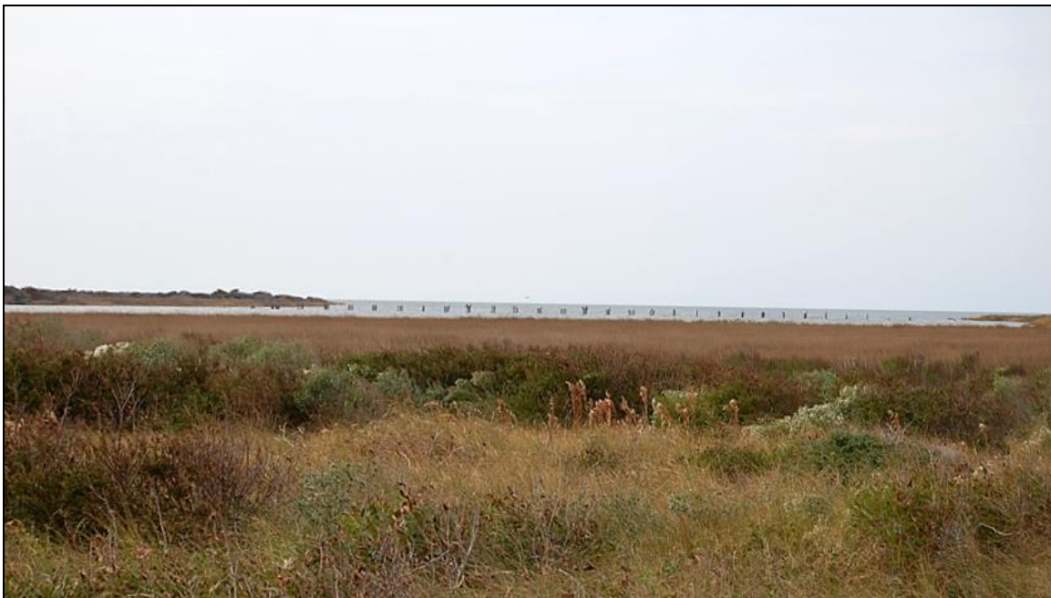
Figure 35. South Channel Bridge from NC 12 (photographer: Marvin Brown, November 9, 2016)
