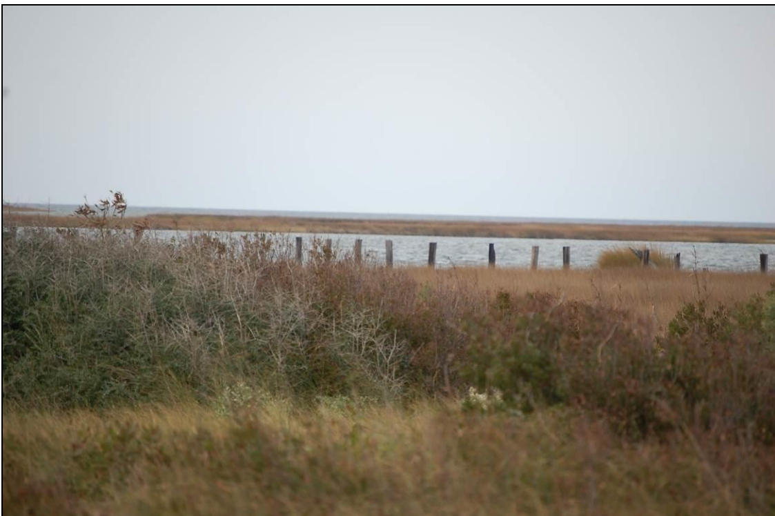
Figure 31. Northern section of North Channel Bridge from NC 12 (photographer: Marvin Brown, November 9, 2016)
