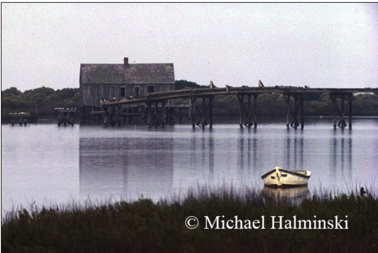
Figure 21. Looking southwest across north channel at bridge and St. Clair Midgett fish camp (photographer: Michael Halminski, 1982)
