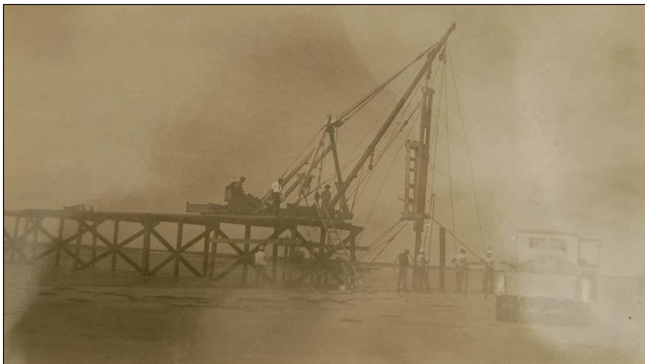
Figure 6. North Channel Bridge: caption reads “Showing Driver across Water of North Channel Sand Beach to Pea Island from here showing Jets at Work” (State Highway Commission, n.d.)
