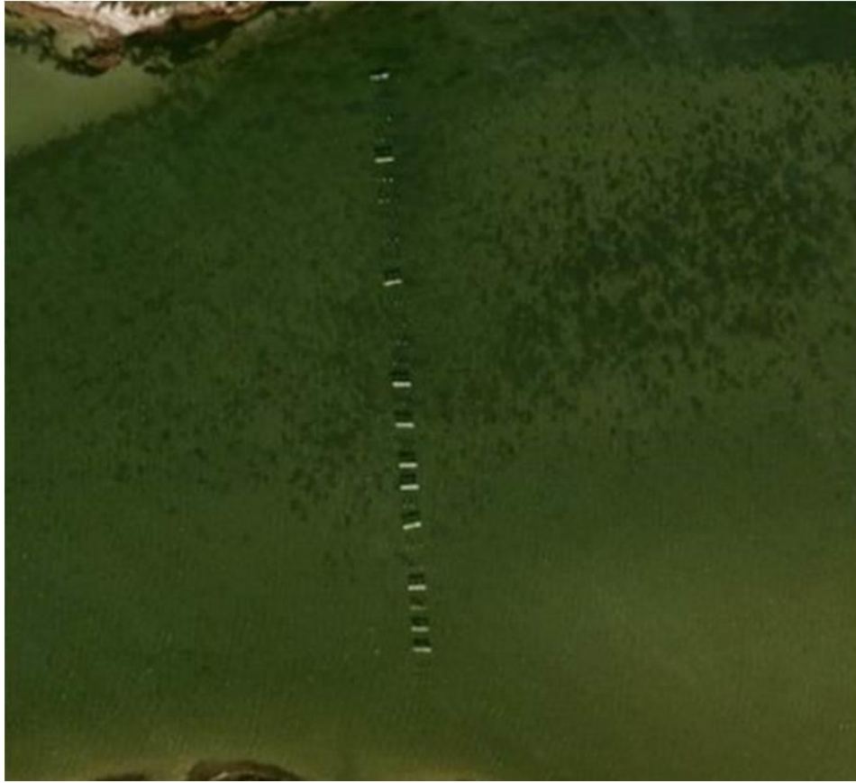
Figure 32. Close up modern aerial view of South Channel Bridge
