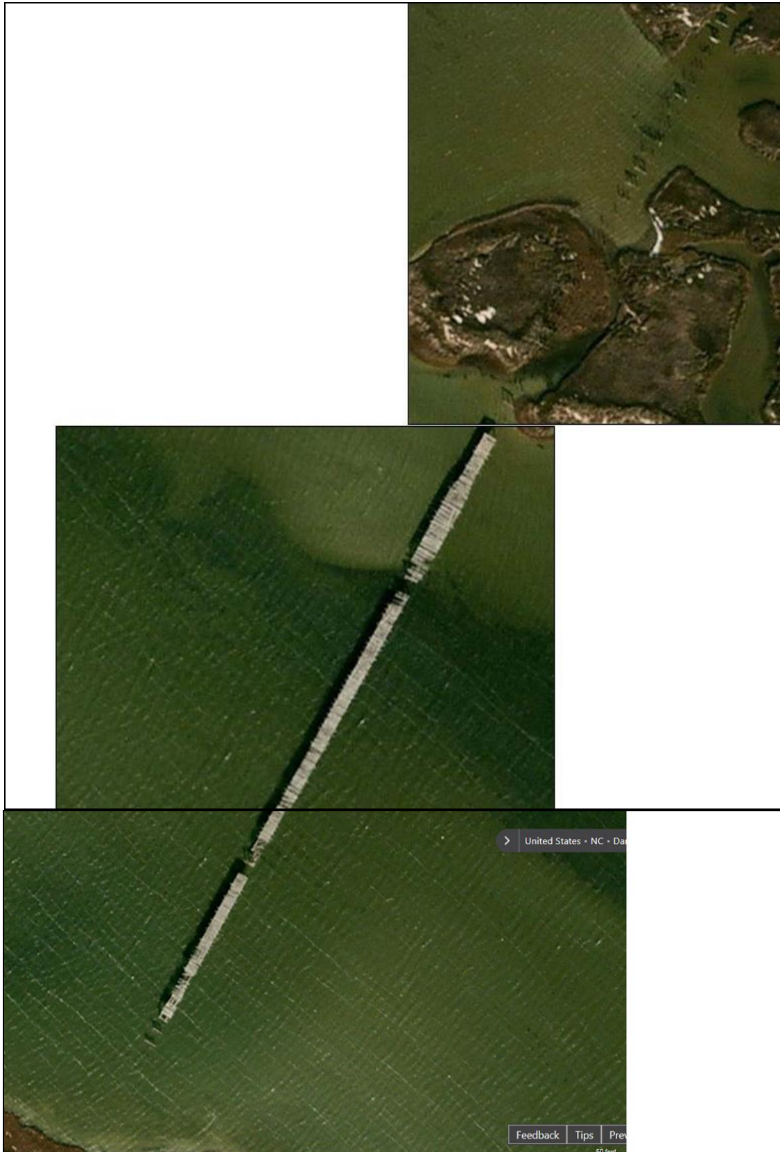
Figure 25. Close up modern aerial view of North Channel Bridge
