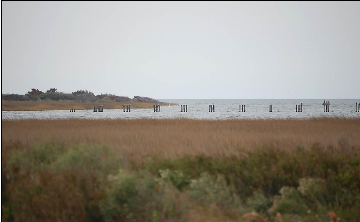
Figure 34. South Channel Bridge from NC 12 (photographer: Marvin Brown, November 9, 2016)
