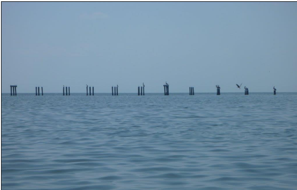
Figure 33. South Channel Bridge from Pamlico Sound (photographer: Dan M. on Panoramio, 2010)
